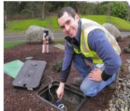
New Meter Installation
